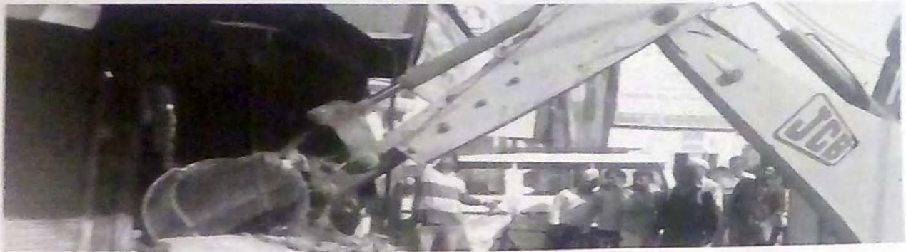
Nagar Palika Parishad, Baraut
